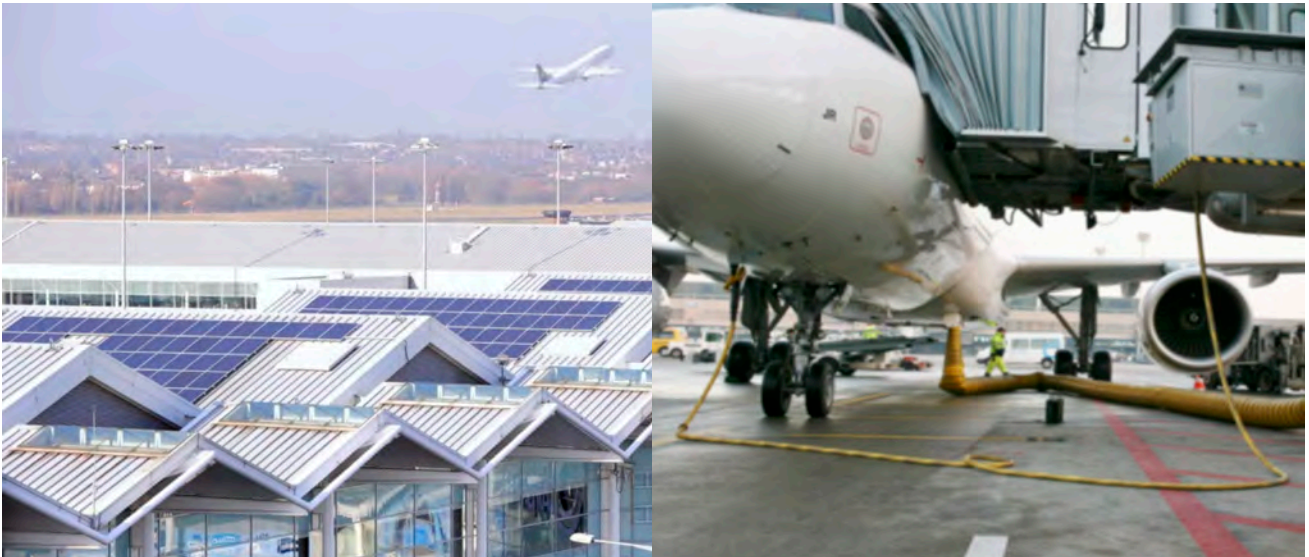
Figure 3. Solar panels at an airport and an aircraft receiving pre-conditioned air and power while parked at a gate. Source: http://www.passengerterminaltoday.com/viewnews.php?NewsID=36516
