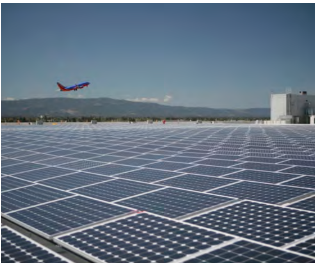
Figure 1. Solar at airport
